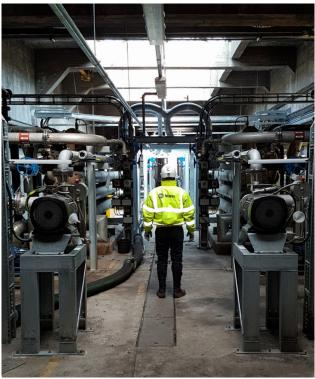
"Since going online in March, April and July last year – four pumps at a time, one on each digester – they've been very good operationally, especially having to work under such duress for those first three months. You could hear them chopping the troublesome filamentous material. From a process perspective, the chopper pump's continuous maceration is very advantageous."
